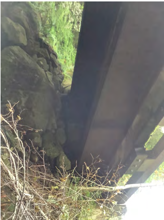
Right Bank Abutment when facing downstream
