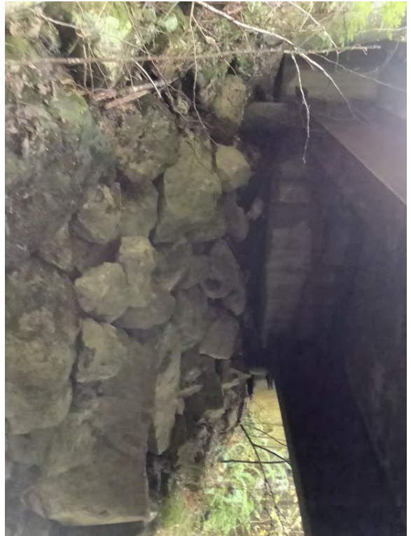
Left Bank Abutment when facing downstream
